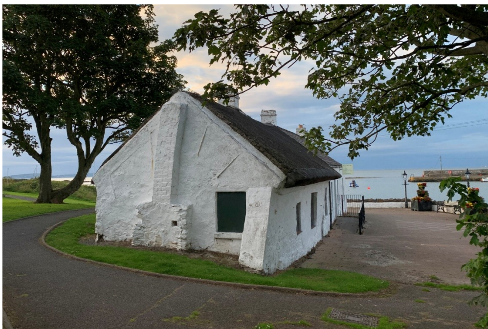
Photo of Cockle Row cottages courtesy of Perry Moore, Groomsport's Generations @ https://www.facebook.com/groups/303870739750690/
